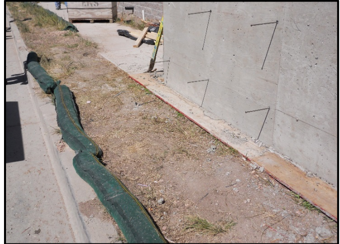
Aggregate Bag used for temporary sediment control
