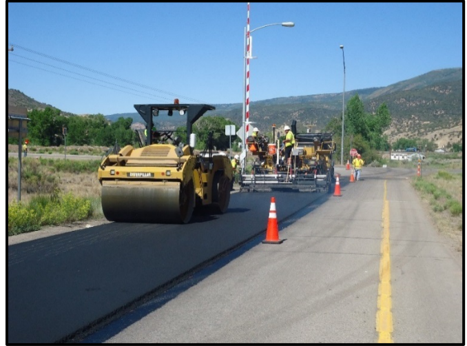
Roadway asphalt paving operations
