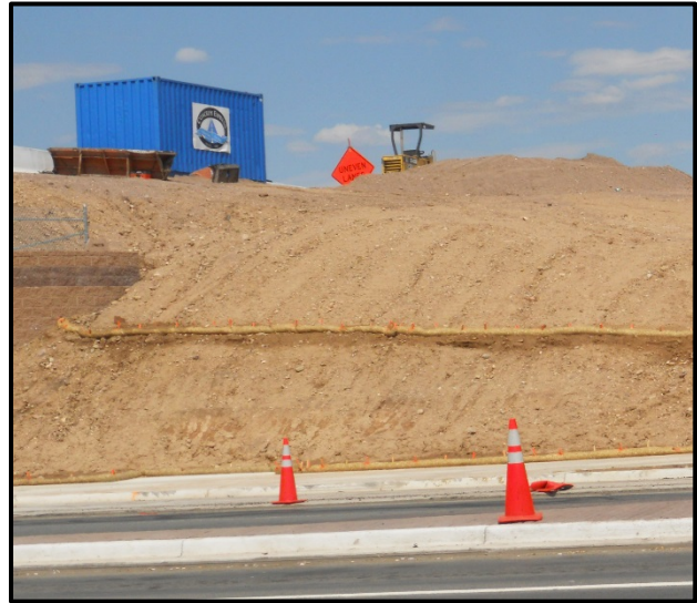
Use of Erosion Logs as temporary slope breaks on disturbed slopes
