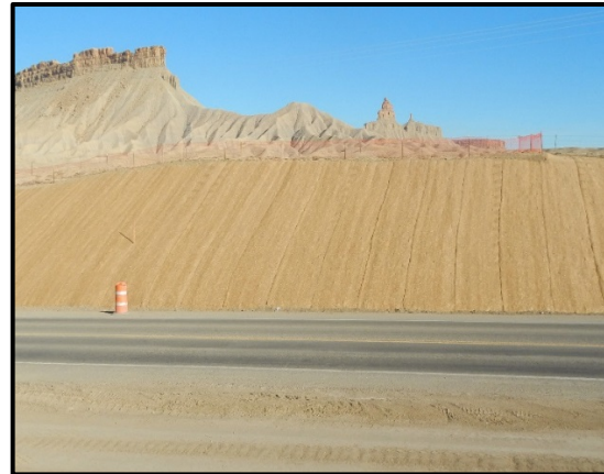
Soil Retention Blanket application on slopes
