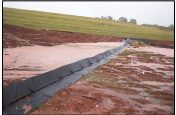
Silt Dike - Credits to South Dakota Department of Transportation
