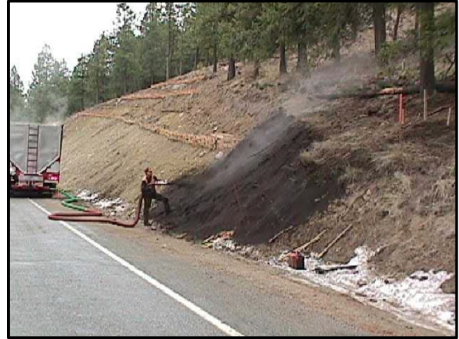
Compost Blanket Applications on Slope
