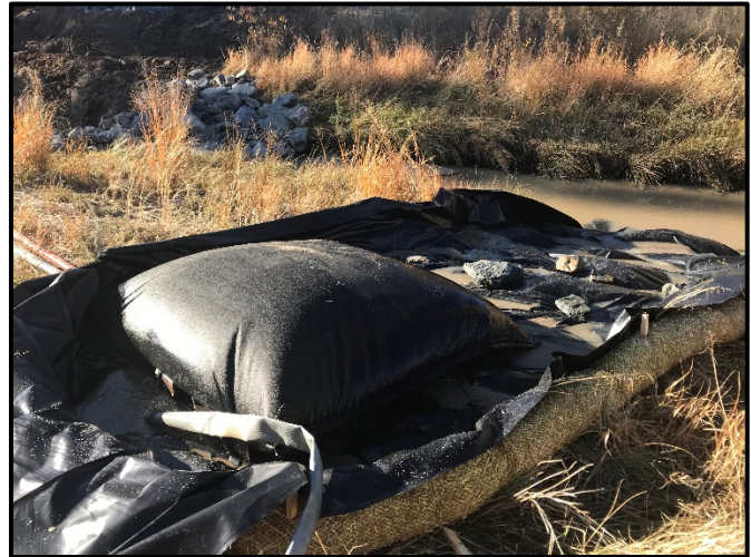
Use of Filter Bag during dewatering operations
