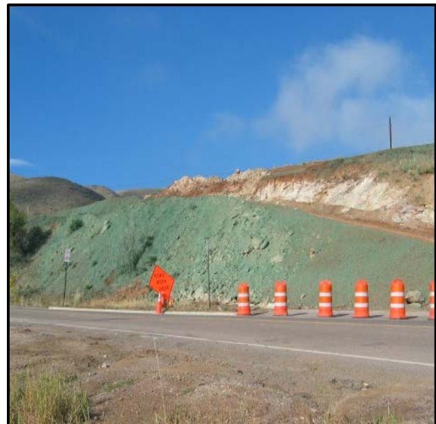
Hydromulch on disturbed side slope
