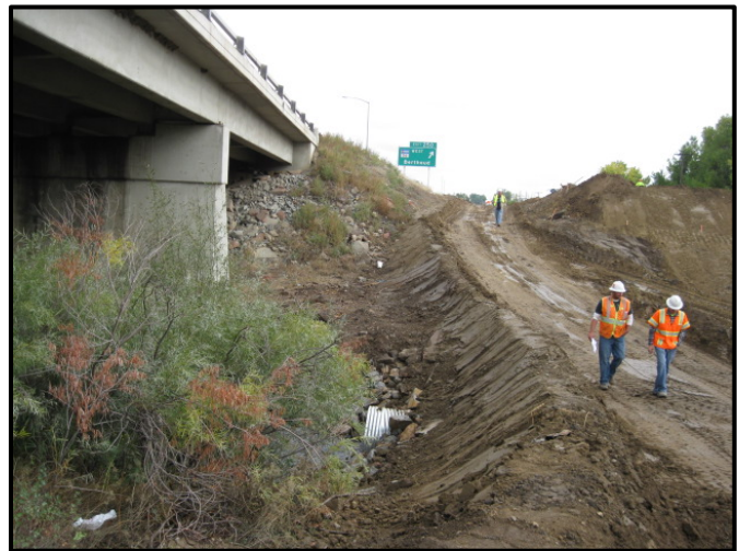
Temporary Berm along access road
