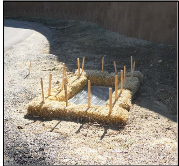
Erosion Bales installation around area inlets
