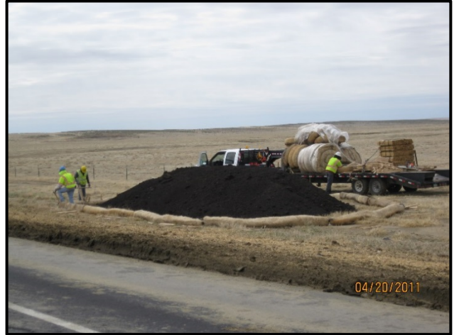
Erosion Logs used for stockpile management practices
