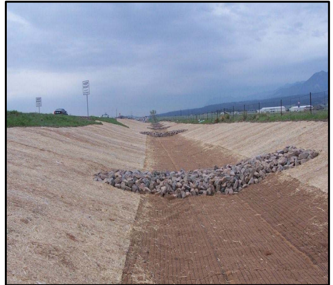
Rock check dam along lined drainage ditch
