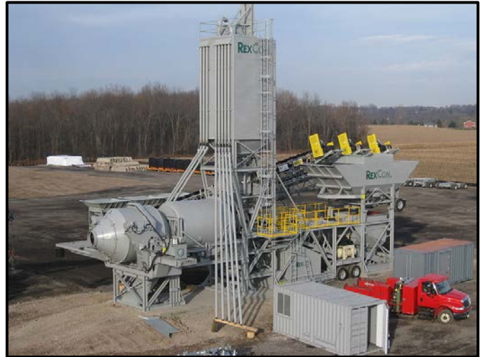
Concrete Batch Plant
